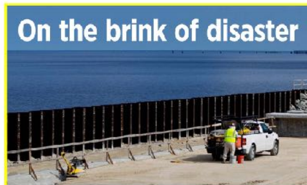
VULNERABLE: Steel wall holds back water from Lake Okeechobee as the Army Corps of Engineers works on the 60-year-old Herbert Hoover Dike. The dike remains on a national shortlist of unsafe Class I dams.
